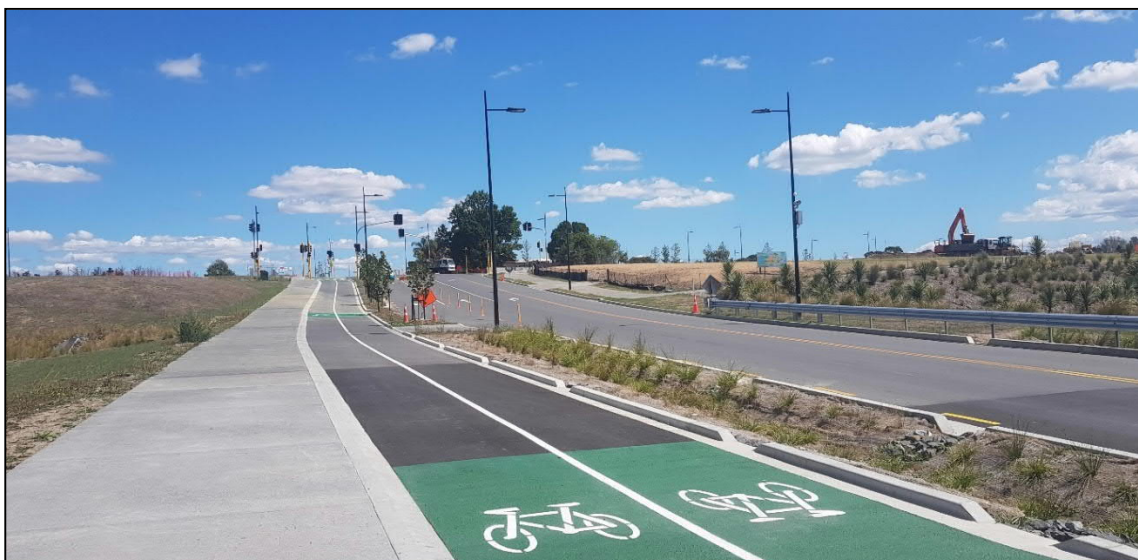
Figure 7-7. Bremner Road upgrade, facing west.
