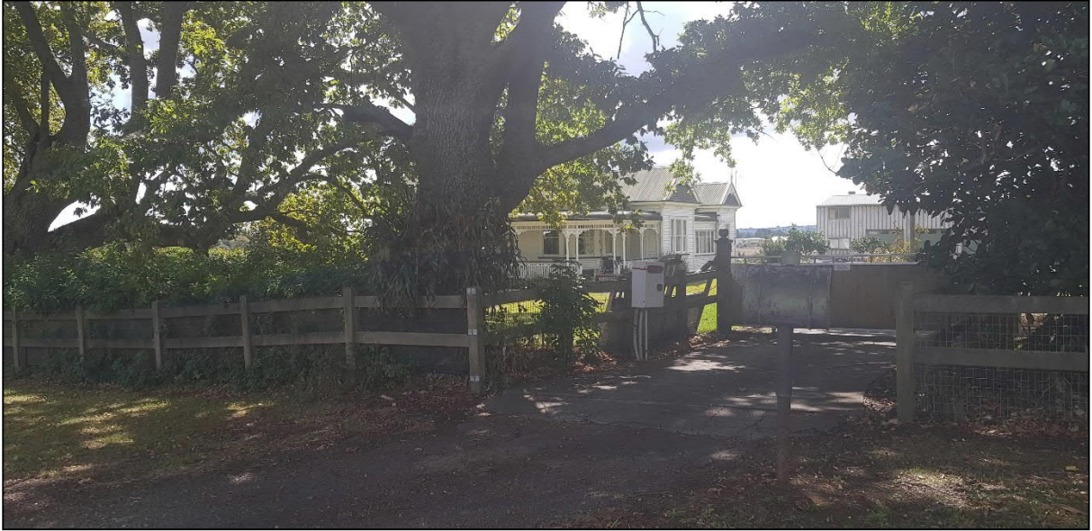
Figure 10-9. Pre-1900s villa (CHI site 22284, R12/1145) facing north (the building is outside of the designation footprint).
