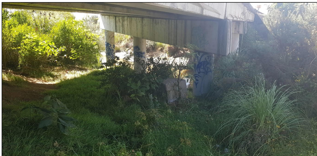
Figure 6-4. Ngakoroa Stream beneath SH22, facing north east
