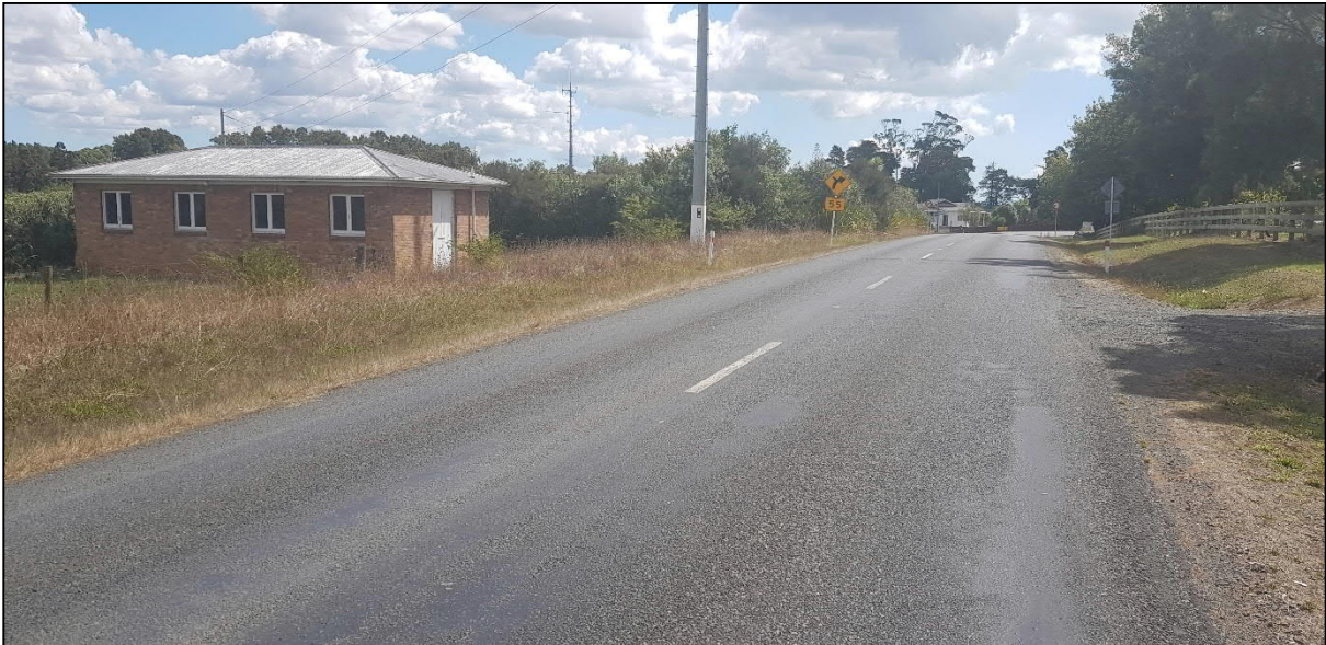
Figure 9-3. The 1940s Utility building, facing west.
