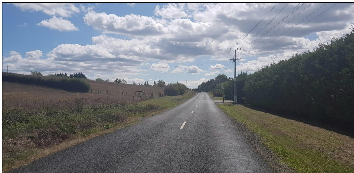
Figure 7-6. View of down Jesmond Road, facing south.
